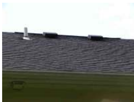
A typical asphalt roof with attic vents
